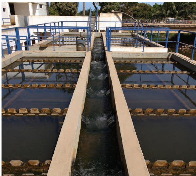
Water supply operations in Angola train workers in maintaining water facilities
