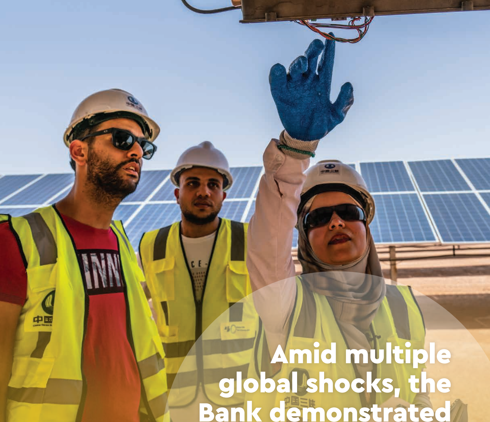
Benban Solar Park in Egypt
